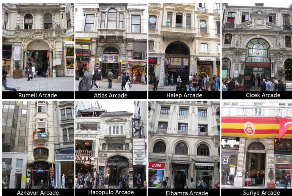
Figure 3: Gates connecting arcades to Istiklal Street
