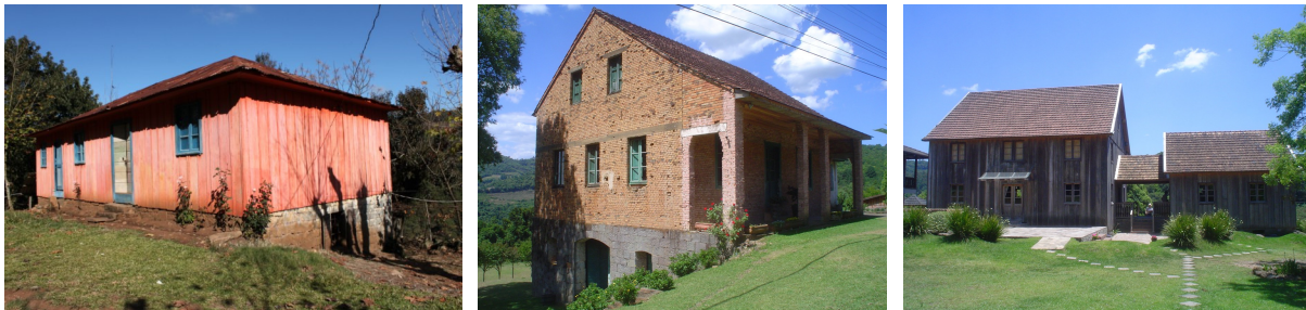
Figure 4: In the left, Somensi House in the Valley, example of a “ feltrina ” house; in the centre, Comioto House, example of a “ bellunese ” house; in the right, House of Pasta, example of a “ ritonda ” house. The authors.
