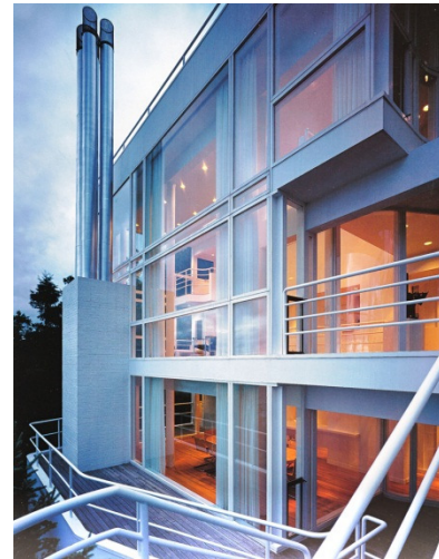
Figure 9: The Western glazed facade showing the white concrete, glass, and stainless steel pipes for the chimney copyright Richard Meier
